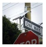
(Left: photo of SFPark.org antenna.) **WiFi transmitters can reach hundreds of feet with just a third of a watt.** Your cell phone can operate with a half- or even a quarter-watt. The older high-power cell phones used to go dead fast because they sucked a lot out of their batteries.
